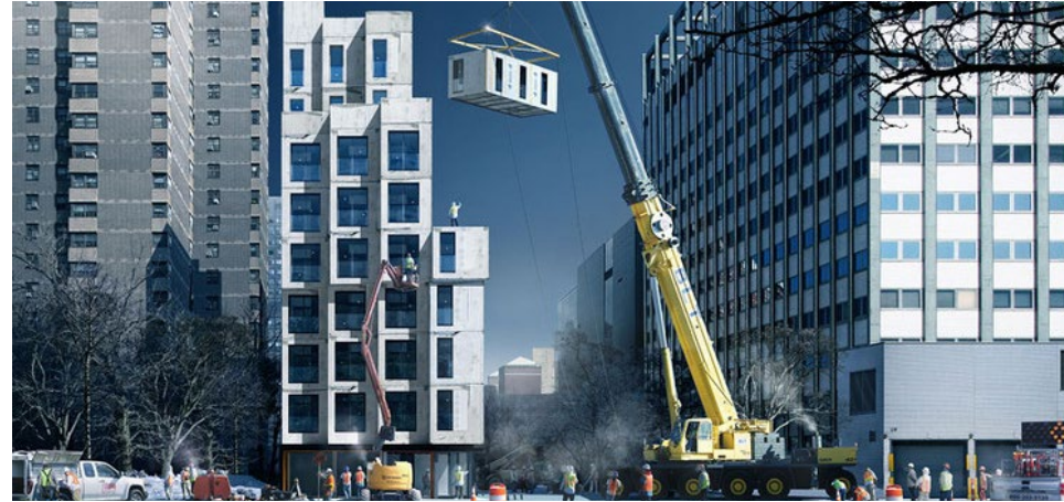
Carmel Place in New York used prefabrication to deliver affordable micro units quickly as part of a pilot project with the city and its housing authority.
