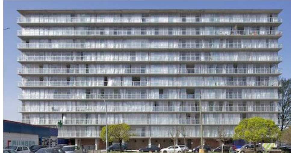
In Bordeaux, France, architects Lacton & Vassal renovated a 1960's era affordable housing block with a new exterior balcony structure. Reinvigorating and maintaining existing buildings is a key to ensuring the availability of affordable housing over time.
