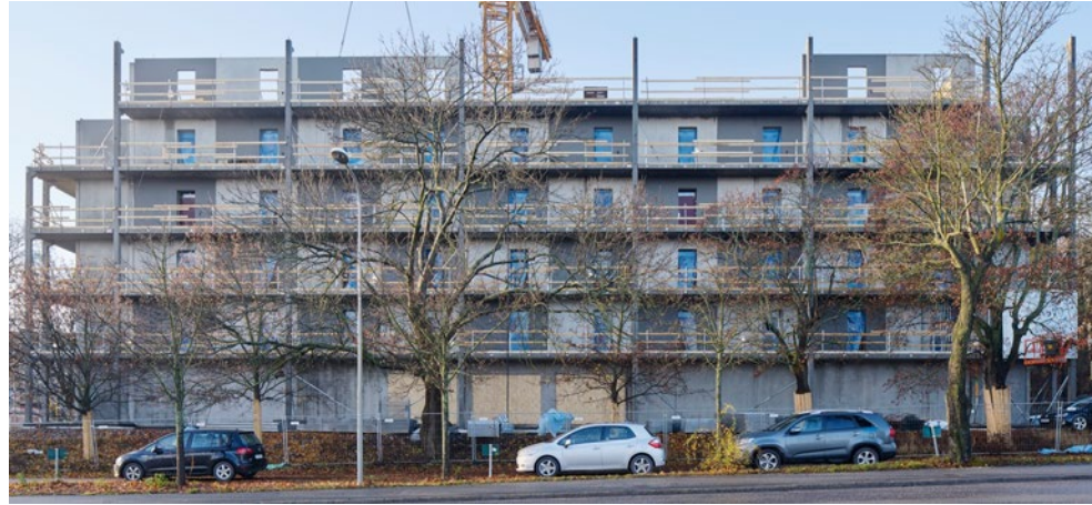
Snabba Hus Vastberga is designed with minimum finishes and standardized materials. The superstructure allows for each modular pre-finished unit to be nested quickly. The interior utilities such as kitchen and washroom are constructed off-site to speed-up delivery.
