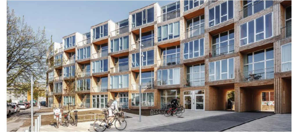
The Dortheavej Residence by Bjarke Ingles Group (BIG) in Copenhagen employs a modular precast concrete system to achieve a unique undulating form.
