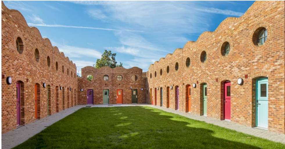
Architect Peter Barber's Holmes Road Studio in London surrounds an open courtyard intended to be developed into a communal garden by the residents.
