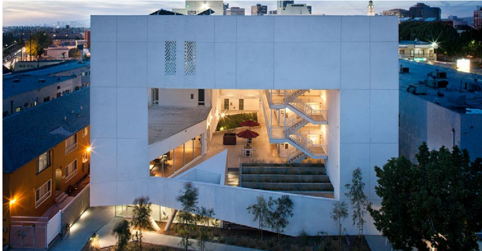
The Six in Los Angeles features supportive housing for homeless veterans. Employing passive design strategies made it 50% more energy efficient than a conventional structure.
