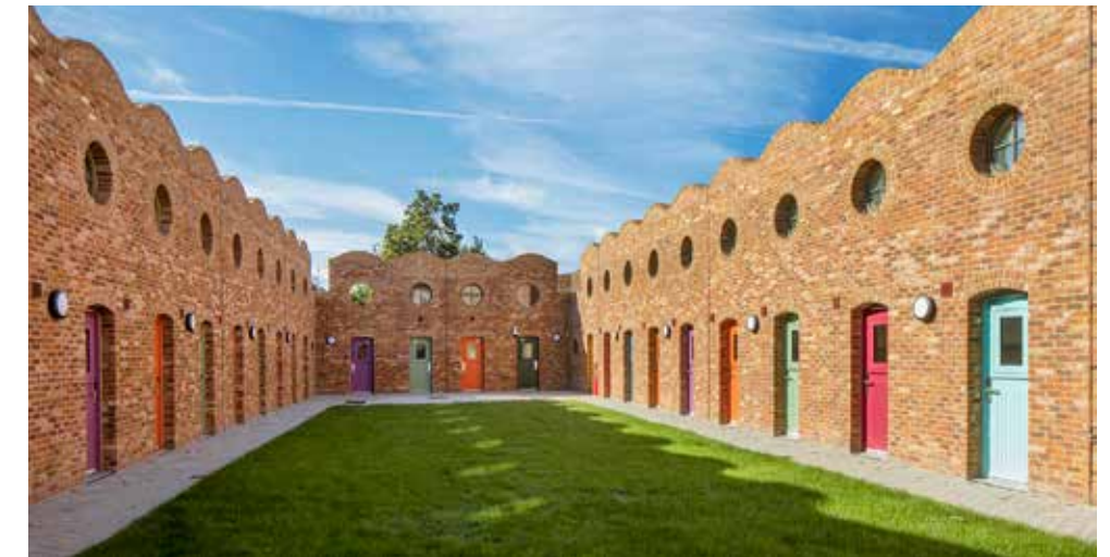
Architect Peter Barber's Holmes Road Studio in London surrounds an open courtyard intended to be developed into a communal garden by the residents.
